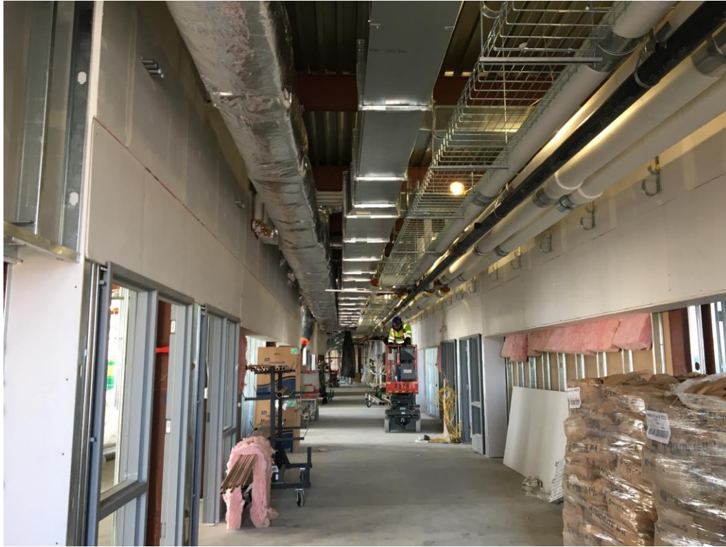
Interior Framing 3 rd Floor (New Addition)
