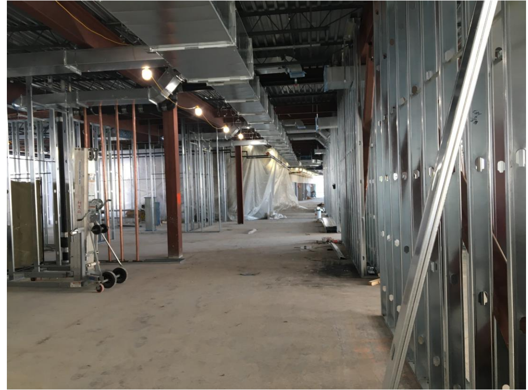
Interior Framing 2 nd Floor (New Addition)
