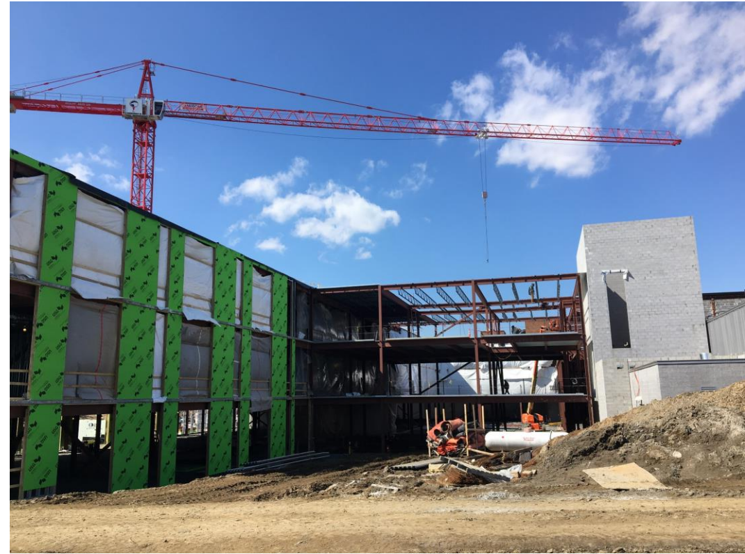
Area 8 & Stair Tower 2-4 (New Addition)
