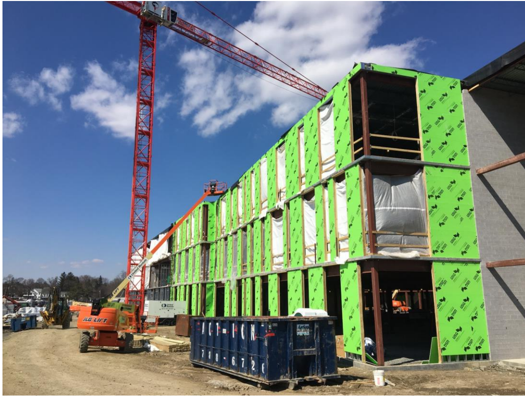
Area 7 & 8 (New Addition)
