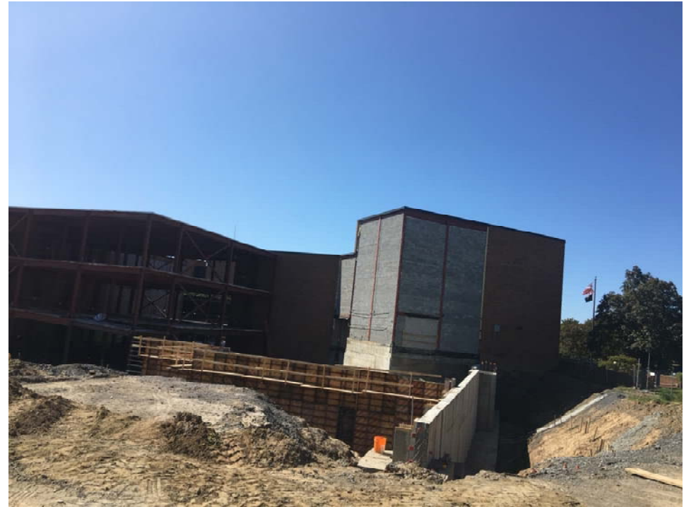
Area 5 (New Addition)
