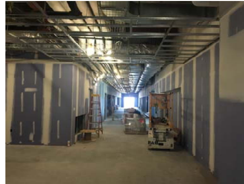
Interior Framing 2 nd Floor
