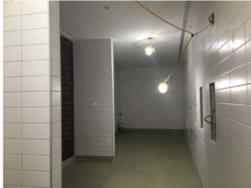
3 rd Floor – Bathroom Finishes
