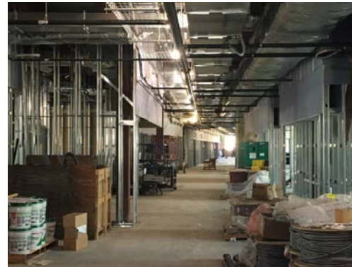
Interior Framing 1 st Floor
