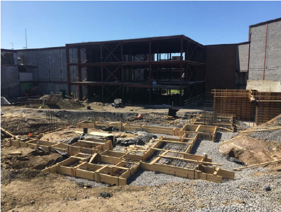
Area 5 (New Addition)
