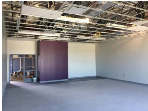
3 rd Floor – Classroom Finishes
